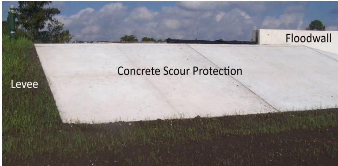
Figure 7 Typical Scour Protection Feature
